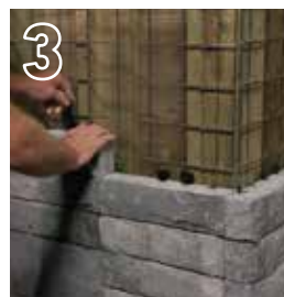
3 Attach Tandem Veneer with Connector
