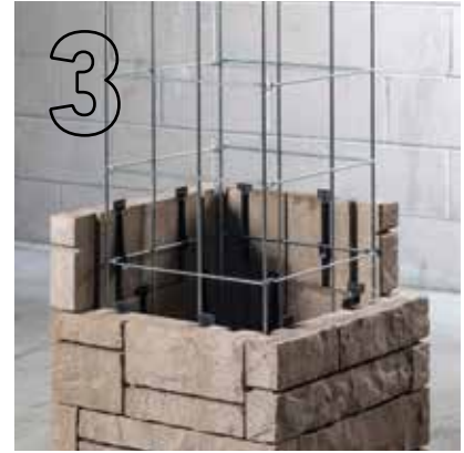
Repeat step 2 and fill with 3/4" crushed rock until column is complete
